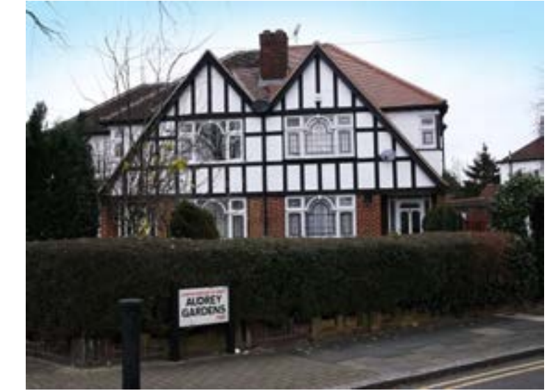
Figure 24: Half timbering at Sudbury Court
